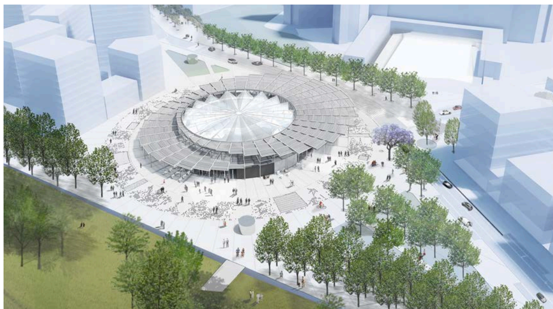
Gare de Villejuif IGR © SGP – Dominique Perrault Architecture
